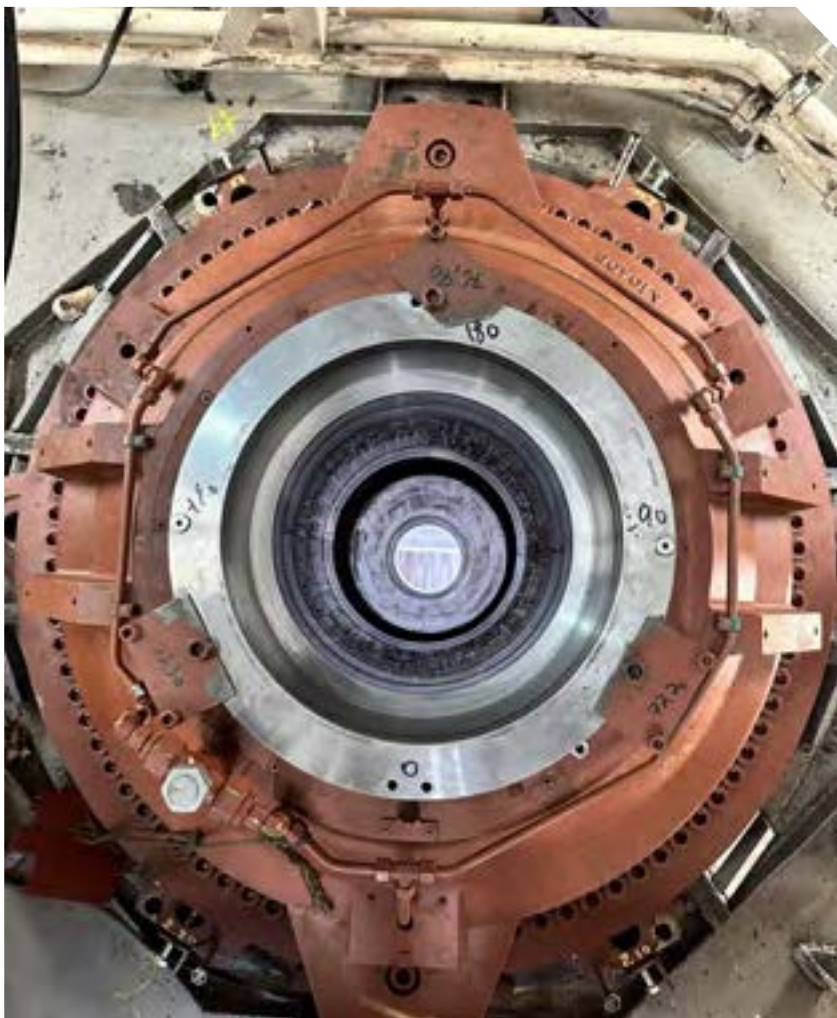
Looking down the rudder line from top of the steering gear – the rudder stock has not yet been reinstalled
