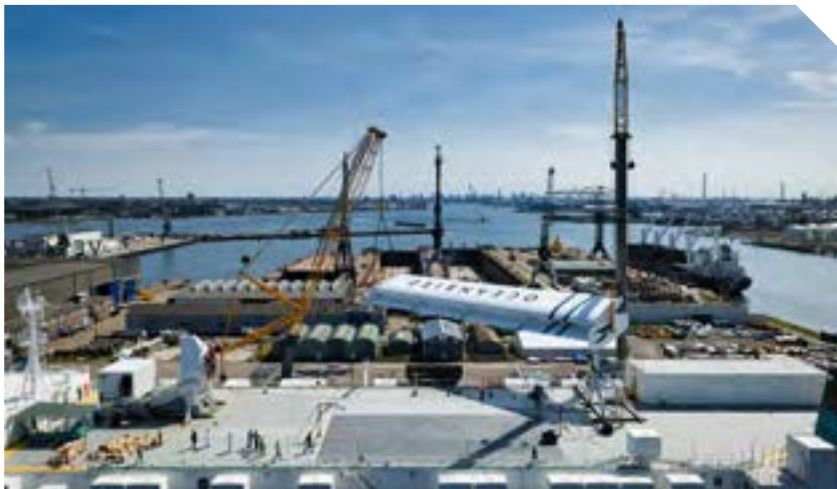
The first installation of an Oceanbird Wing 560
