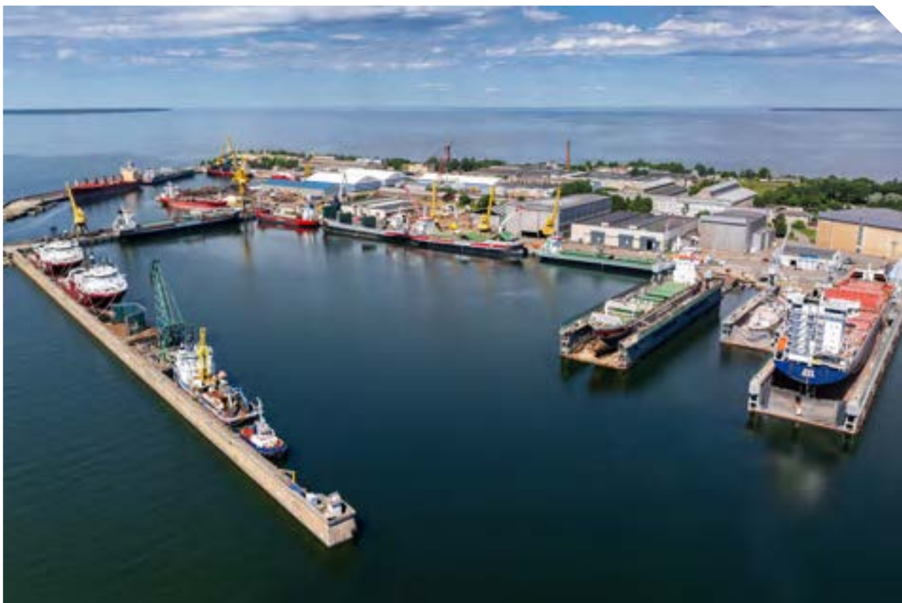
BLRT Repair Yards Tallinn in Estonia
