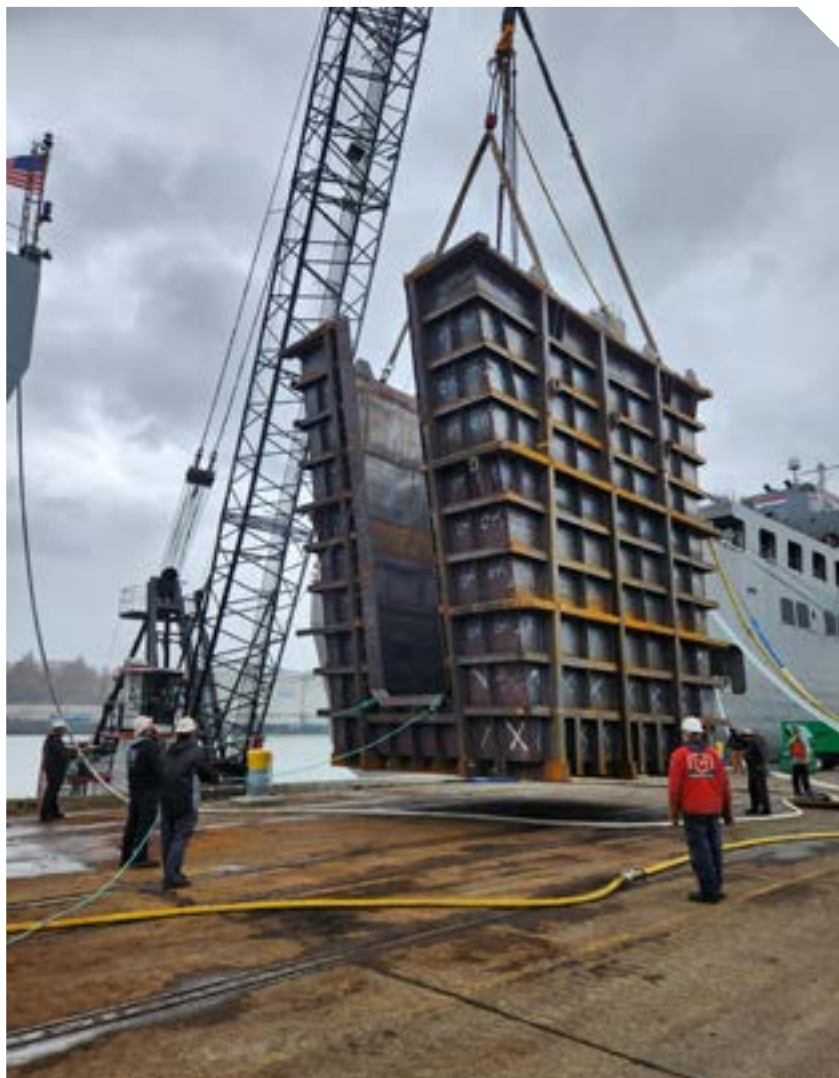
Lifting cofferdam for installation
